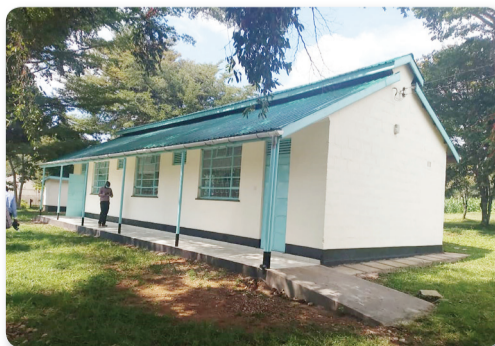
Renovated hall at Miyare ATC.
