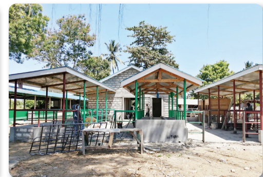
Construction of a Dairy Unit at Mtwapa ATC
