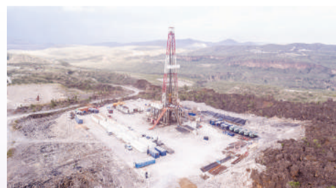
KenGen Geothermal Drilling Rig at Olkaria. KenGen currently supplies about 72% of the electricity consumed in Kenya, with 86% of this coming from renewable and clean energy sources.
