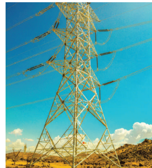
A tower in a section of the 400kV Loiyangalani - Suswa Transmission Line.
