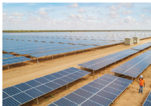
The 50 MW Garissa Solar Power Plant.
