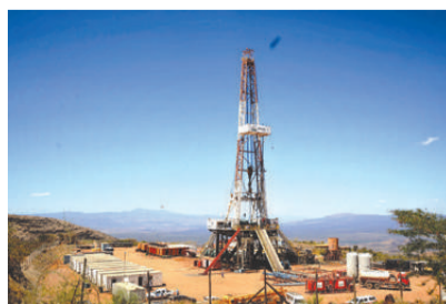
A rig in the Korosi Prospect, Baringo – Silali project
